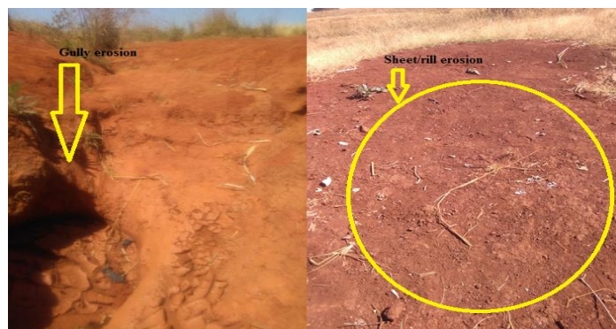
Figure 6: A plate showing a sign of soil erosion at western block (Amba 16 kebele)
